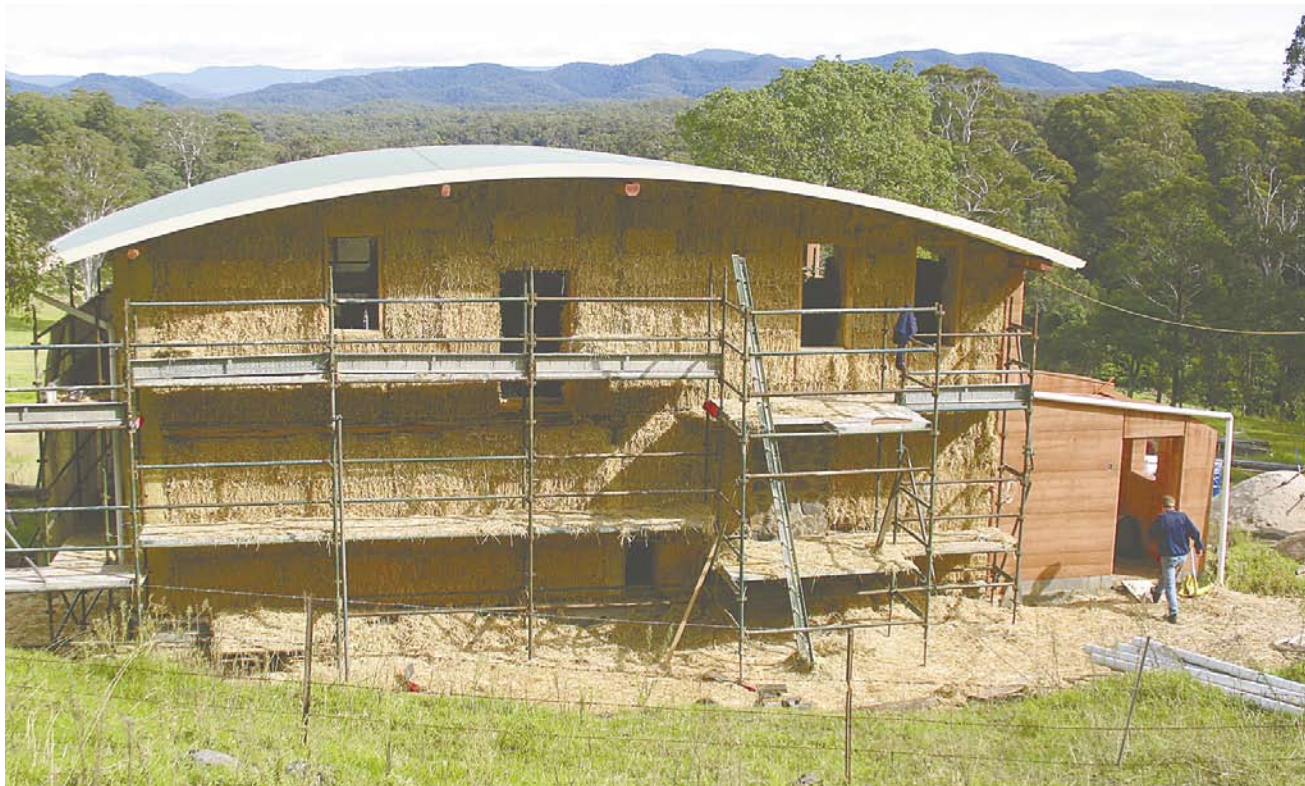
At the completion of the four-day workshop, the walls had all been raised and we were ready to start the render.
