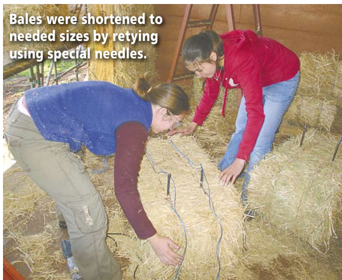
Bales should be aligned before tying down.
